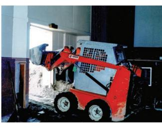
Above: Inside Floor.... The auditorium flooring was replaced removed and concreted in 2005. Photo: OCN
